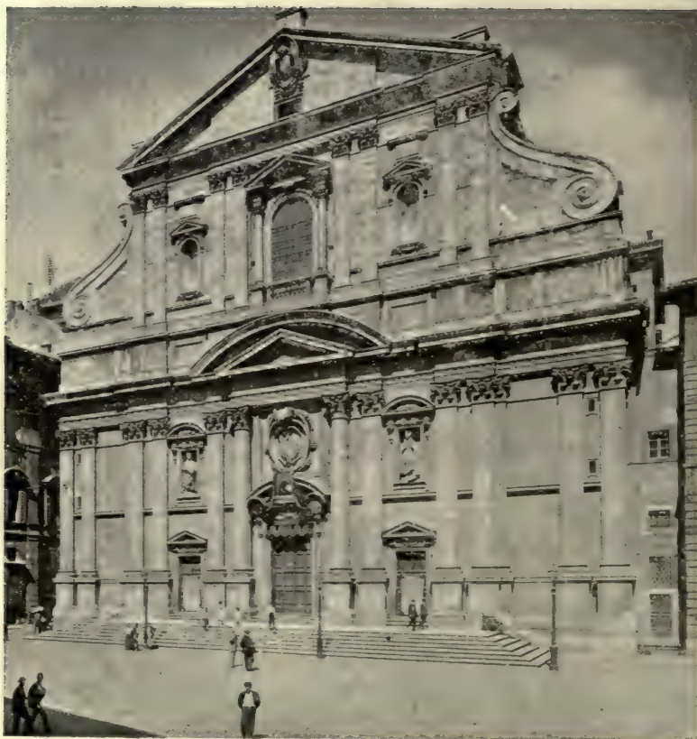
FAÇADE Church of the Gesù, Rome
